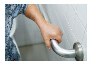
Vertical rails can assist people when pulling up from a seated position or walking up a single step.
